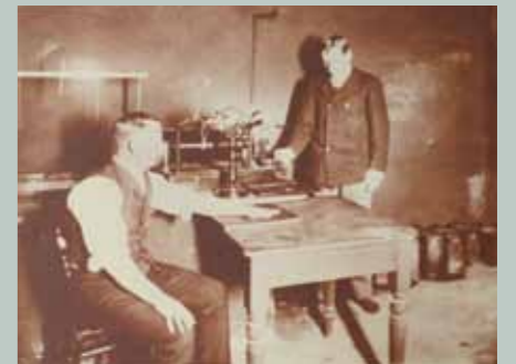
Newly installed X-ray department in the lower ground floor, around 1902.
